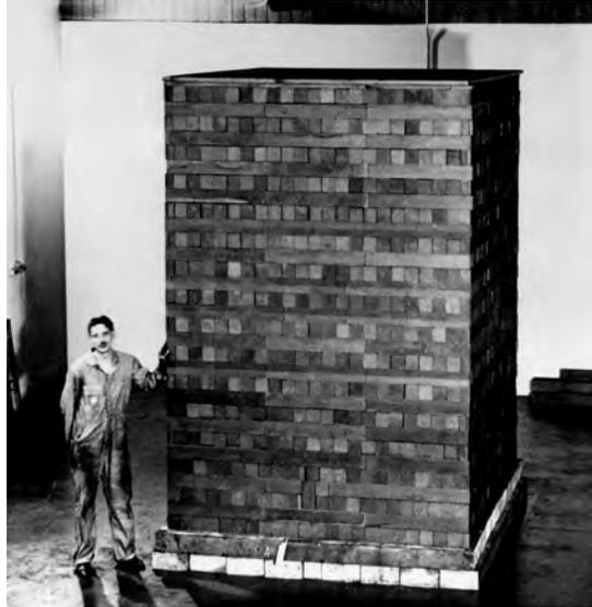
**Fig. 2.** Likely an early exponential pile. If the man is about five feet tall, this was probably an 8 by 8 by 11-foot exponential pile. *Source:* <https://www.atomicheritage.org/history/chicago-pile-1>
