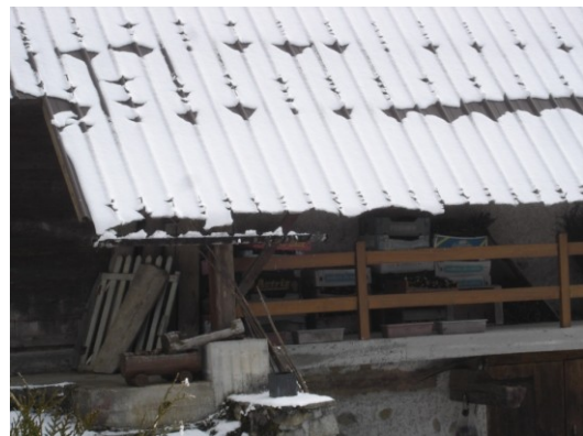
Fig 2: Incipient wet snow full-depth avalanche on a barn roof. Numerous crown cracks open at every weak place, due to low rupture stresses of wet snow. Note the limited lateral extension of such cracks, related to low yield stresses that favour easy blunting (see text). Some of them may merge (on the right) giving large cracks that may trigger the avalanche.
