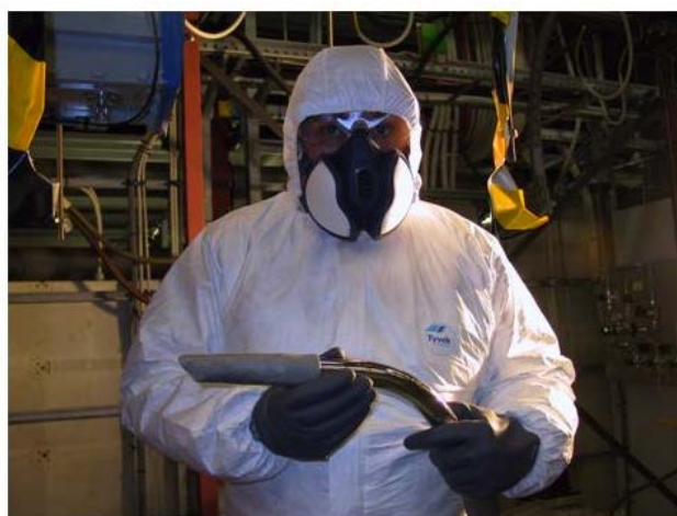
Fig. 9: Staff wearing protective clothing during work with SF 6 waveguides
