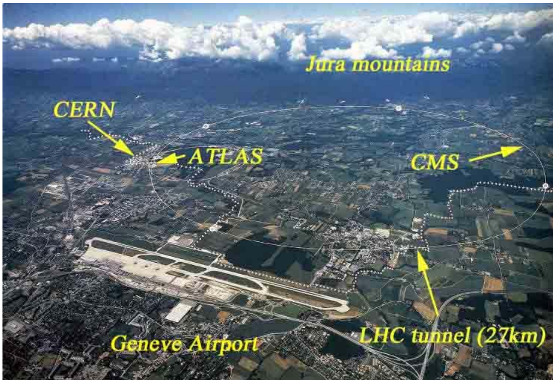
Figure 7. The LHC tunnel, detectors, and the Jura.
