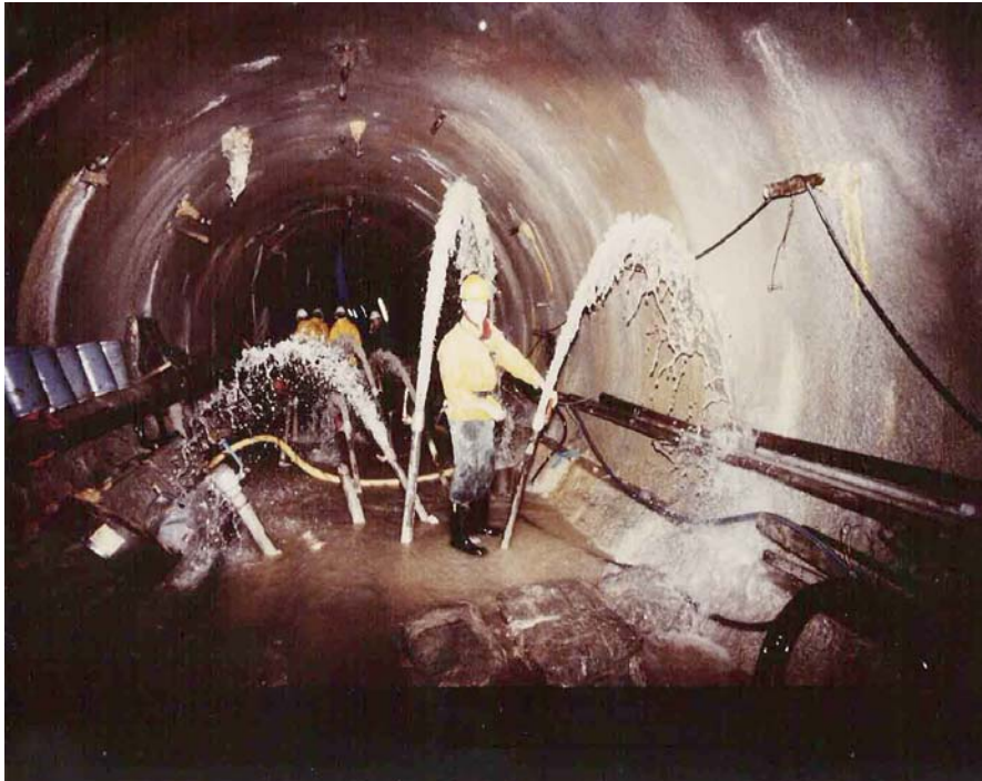
Figure 6. LEP tunnel water in the Jura region.
