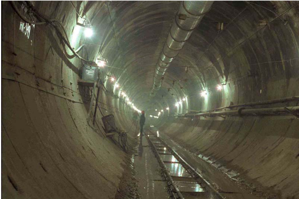
Figure 4, The UNK tunnel under construction
